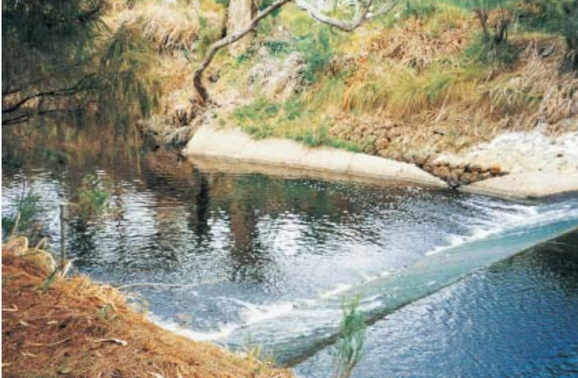
Weirs such as this one restrict flow and bank up water in times of low flow. In this case, when the river has been flowing quickly erosion has resulted in engineering works being required to protect the bank. Photo Siwan Lovett.
