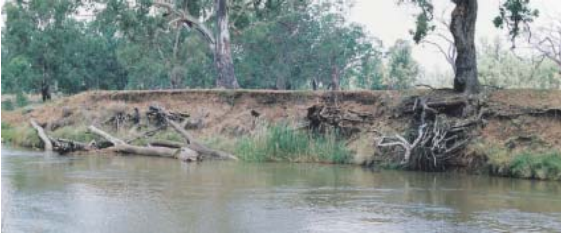
The grasses, reeds, logs and branches at the toe of this bank are protecting it against further erosion. The site would respond well to rehabilitation as the toe is currently protected and there are some trees remaining on the riverbank to help bind the soil and provide a seed source for regeneration. Photo Guy Roth.
