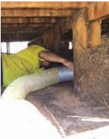
The long suction tube can extend 50m and reach confined and restricted areas.
