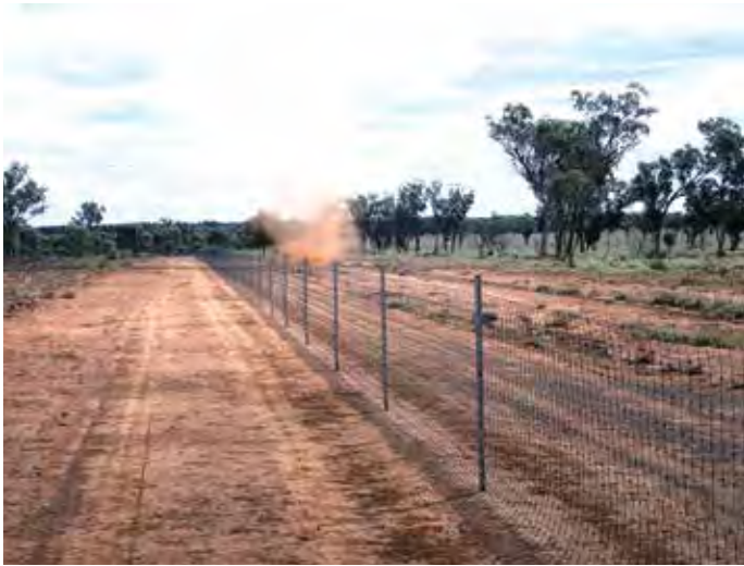
Prefabricated wire with a fixed footer (preferred fencing for Queensland cluster fences).
