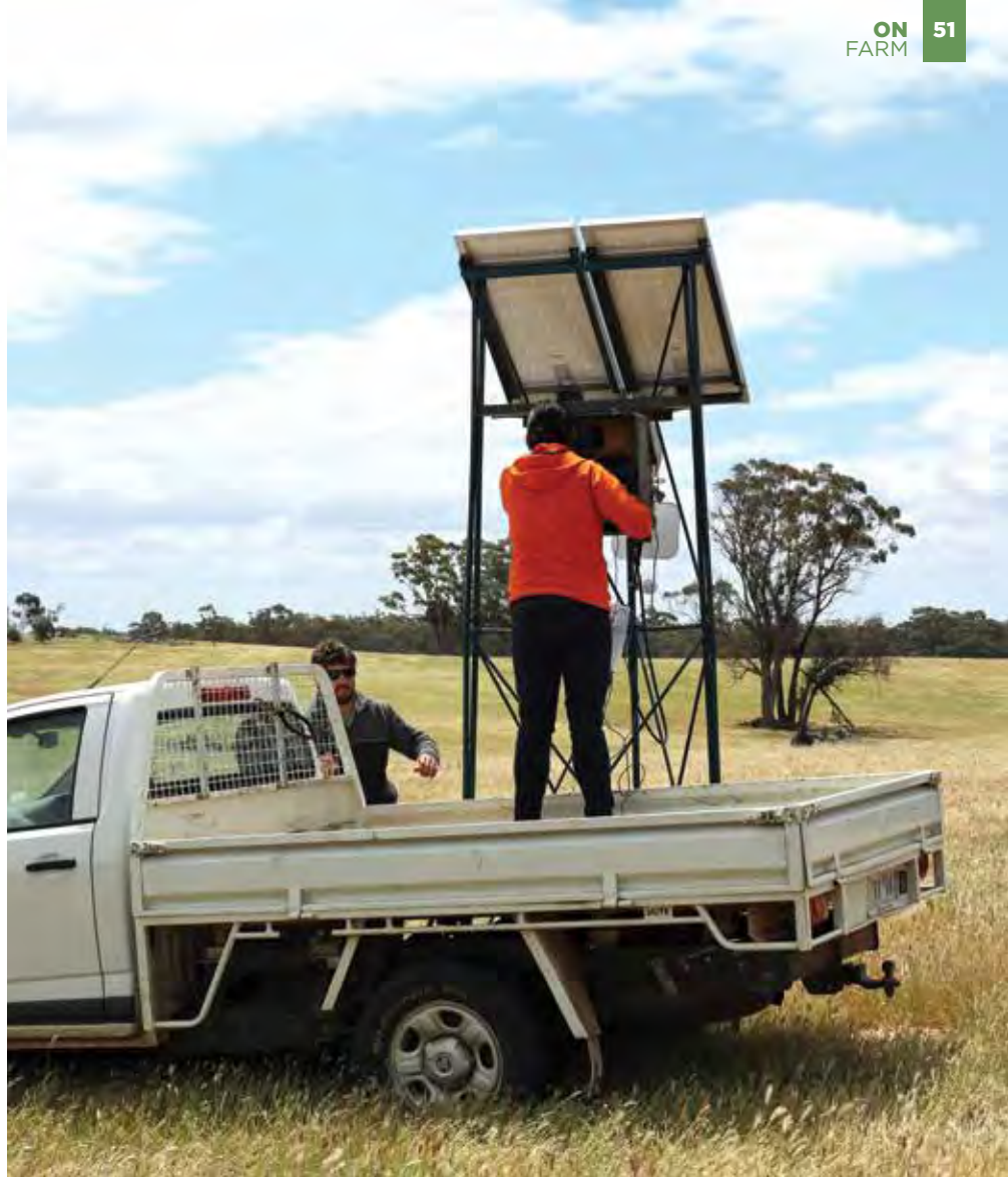
Installing a solar powered wireless antenna on Tony Butler's property.
