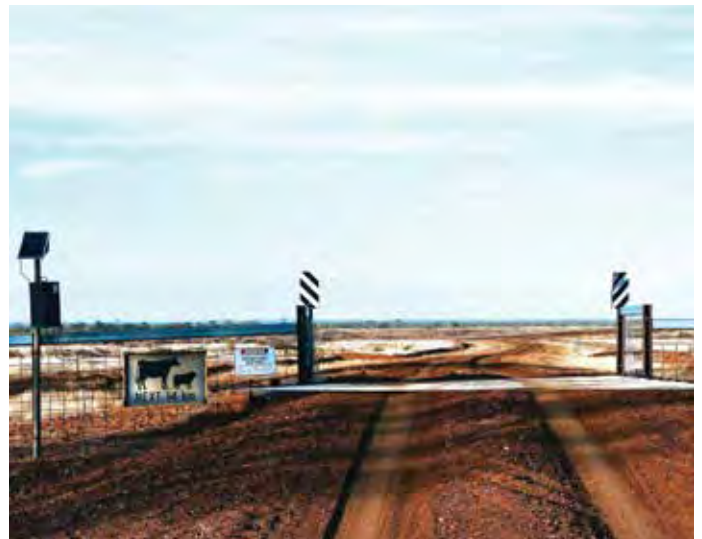
Electrified tape being used to prevent wild dogs negotiating grids. The tape is electrified using a solar-powered energiser . This grid also incorporates a motion-activated light and siren to deter wild dogs.
