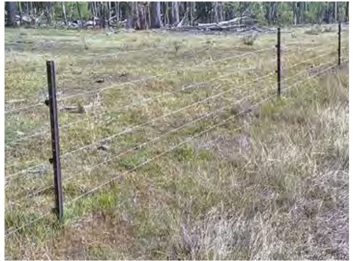
Plain electric wire fence with an electrified ground/bottom wire (often used in hilly terrain, for example eastern Victoria).
