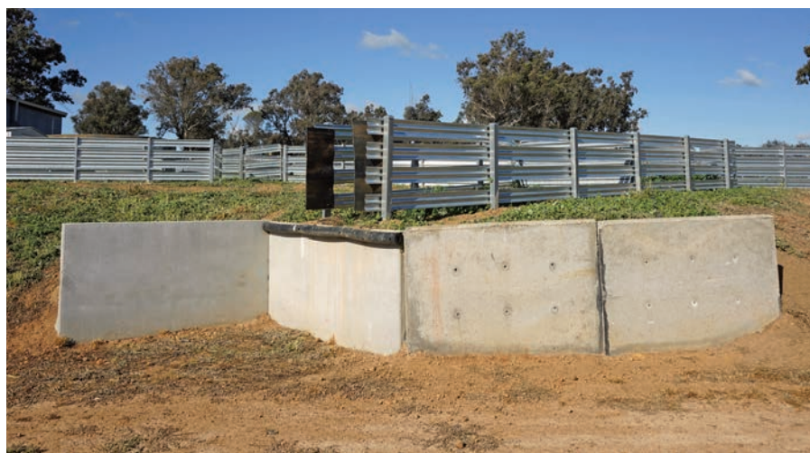
Loading ramp utilises the site slope.
