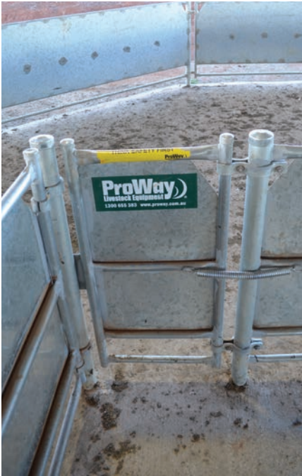
Personal Access gate.
