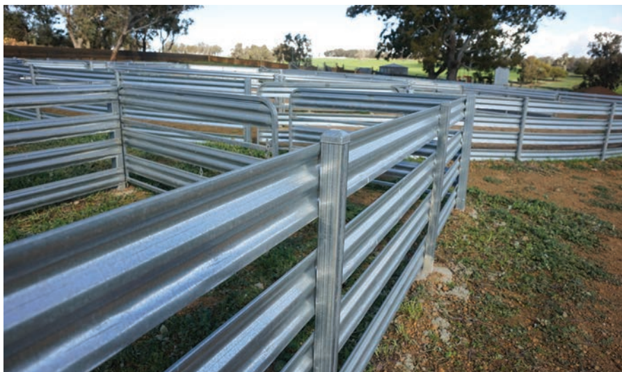
75mm SHS posts and K-rail style panelling.
