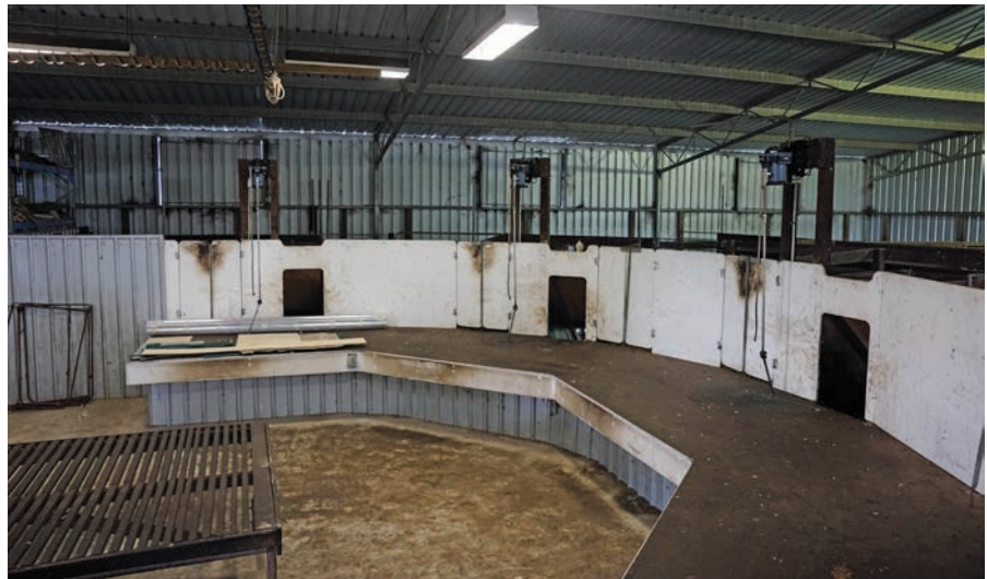
Horseshoe raised board shearing shed.
