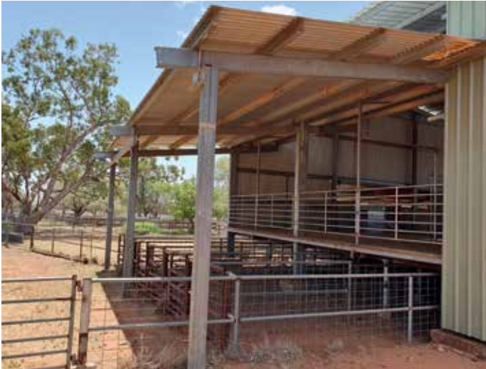
Figure 14: steel structural beams and covered count out pens.
