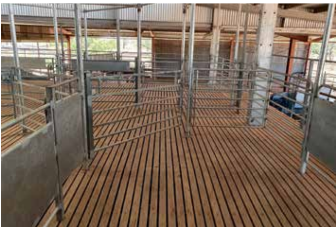
Figure 8: shows the in-shed yards, slide/swing gates and boarded catching pen fence panels.
