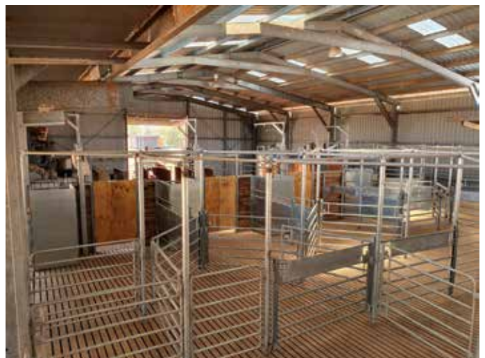
Figure 9: the timber slats in the catching pens run towards the board, parallel to the drag path. Where they are running against the flow of sheep in the rest of the back pens to reduce vision/light from underneath as sheep are penned up.
