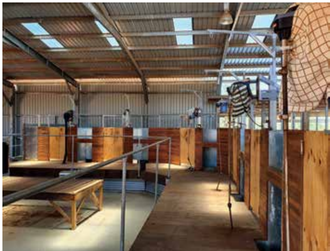
Figure 11: right angle board design, with a raised rail to reduce the fall hazard. Note the electric shearing plant are covered while not in use.
