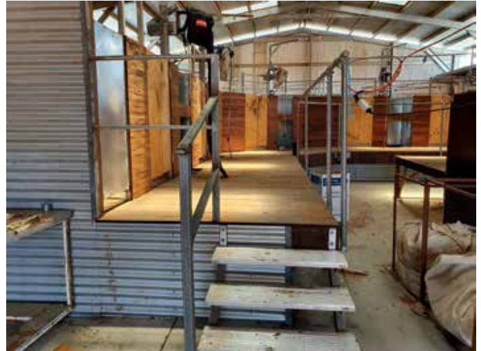
Figure 12: showing the concrete wool room floor and the stairs which are fixed to the raised board with a handrail.
