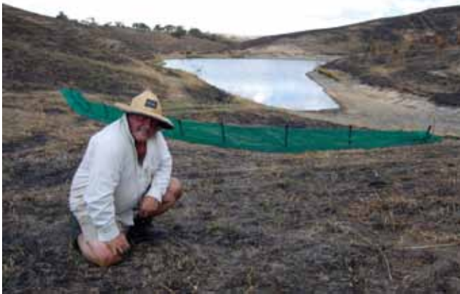
Figure 5.1: Sediment fence built to protect dam from debris and pollution after fire.
