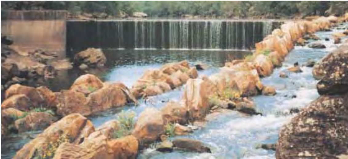
This weir has had a rock ramp fishway built alongside so that native fish can continue to move up and down the river, something which many of the diversions and barriers along our rivers has prevented. Photo Stuart Blanch.
