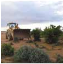
Figure 2 Removal of Box Thorns
