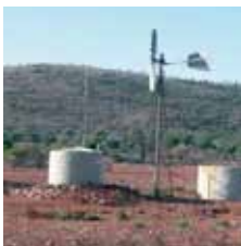
Figure 4 The system works effectively even on distant waters surrounded by difficult terrain.
