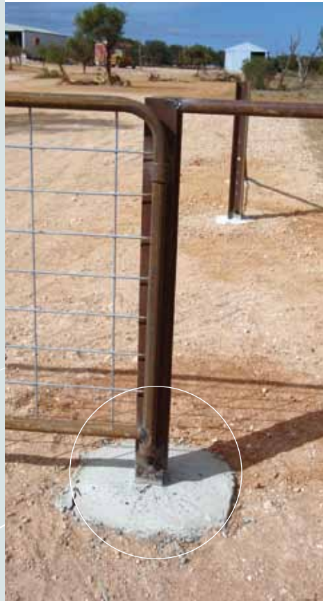
Figure 1 Inverted hinge system
