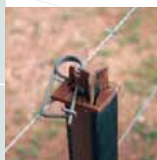
Figure 2 Cotter pin holding the sleeve onto the dropper
