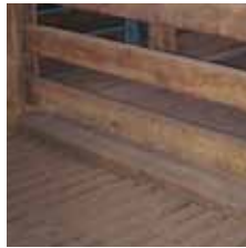
Figure 2 Declining slope of floor to the front of catching pens for ease of drag
