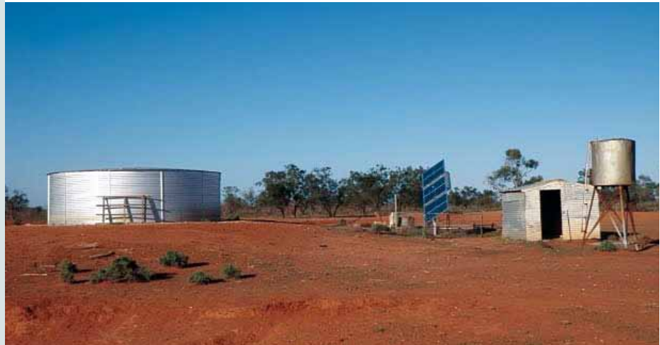
Figure 1 Solar pump and new tank
