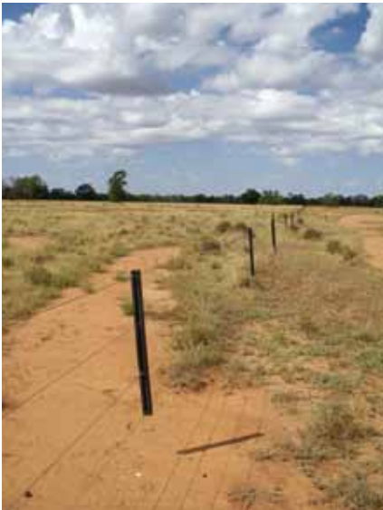
Figure 2 Four plain wires running through Westonfence droppers
