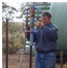
Figure 2 Using the Marchant Picket Post Driver to drive in droppers
