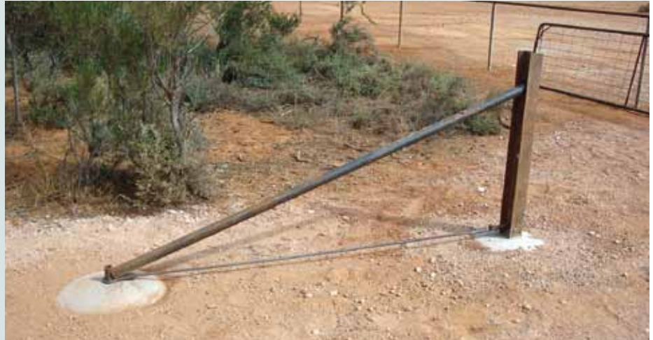
Figure 1 The new strainer system
