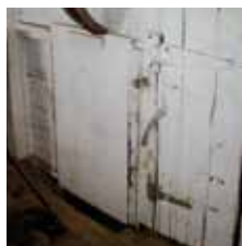
Figure 4 Vertically sliding doors to cover the chute when not in use
