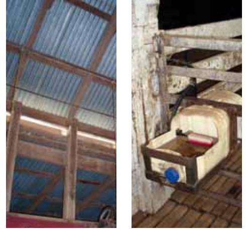
Figure 7 Purpose built water troughs in the large holding pens
