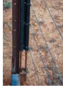
Figure 4 Weston fencing system using a slide attached to the dropper
