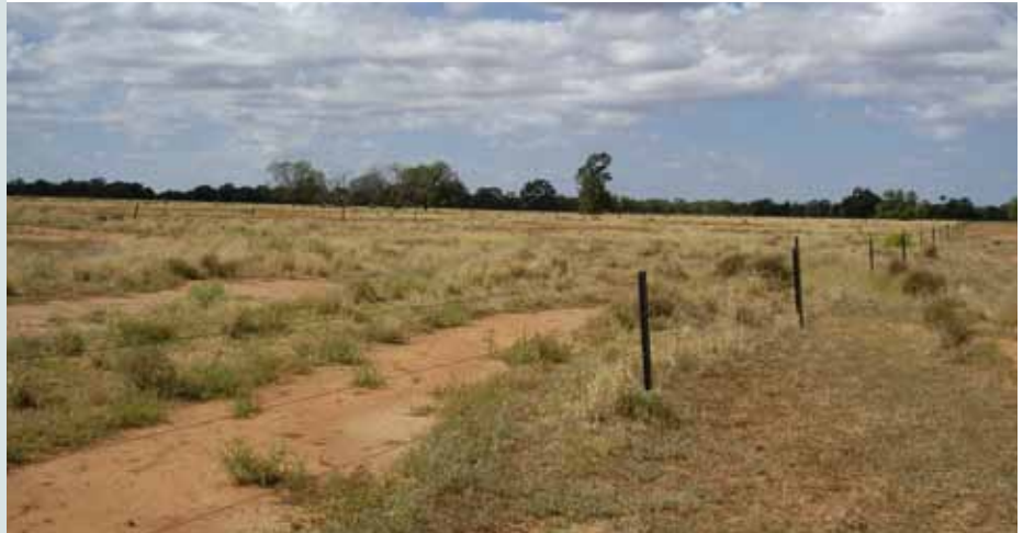
Figure 1 13km electric laneway
