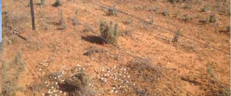
Figure 5: Spirals are used to attach the short length of fence to the raised fence.
