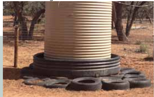
Figure 3: Cup and saucer trough with tyres at the base to mitigate erosion.
