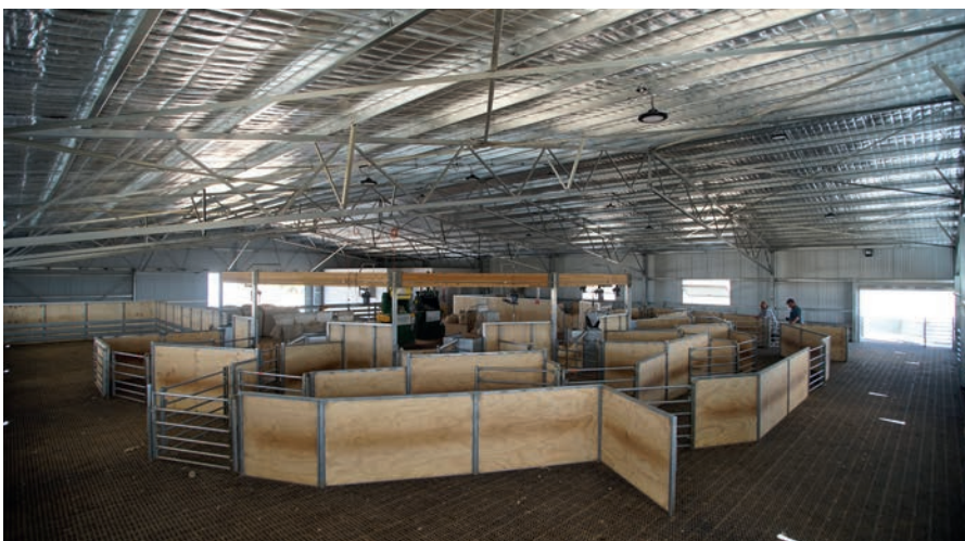
Plyable: Use of marine ply is a signature feature of Chippy Chad & Co shed fitouts but the Bilney shed extends the use into the sloped catching and holding pens.
