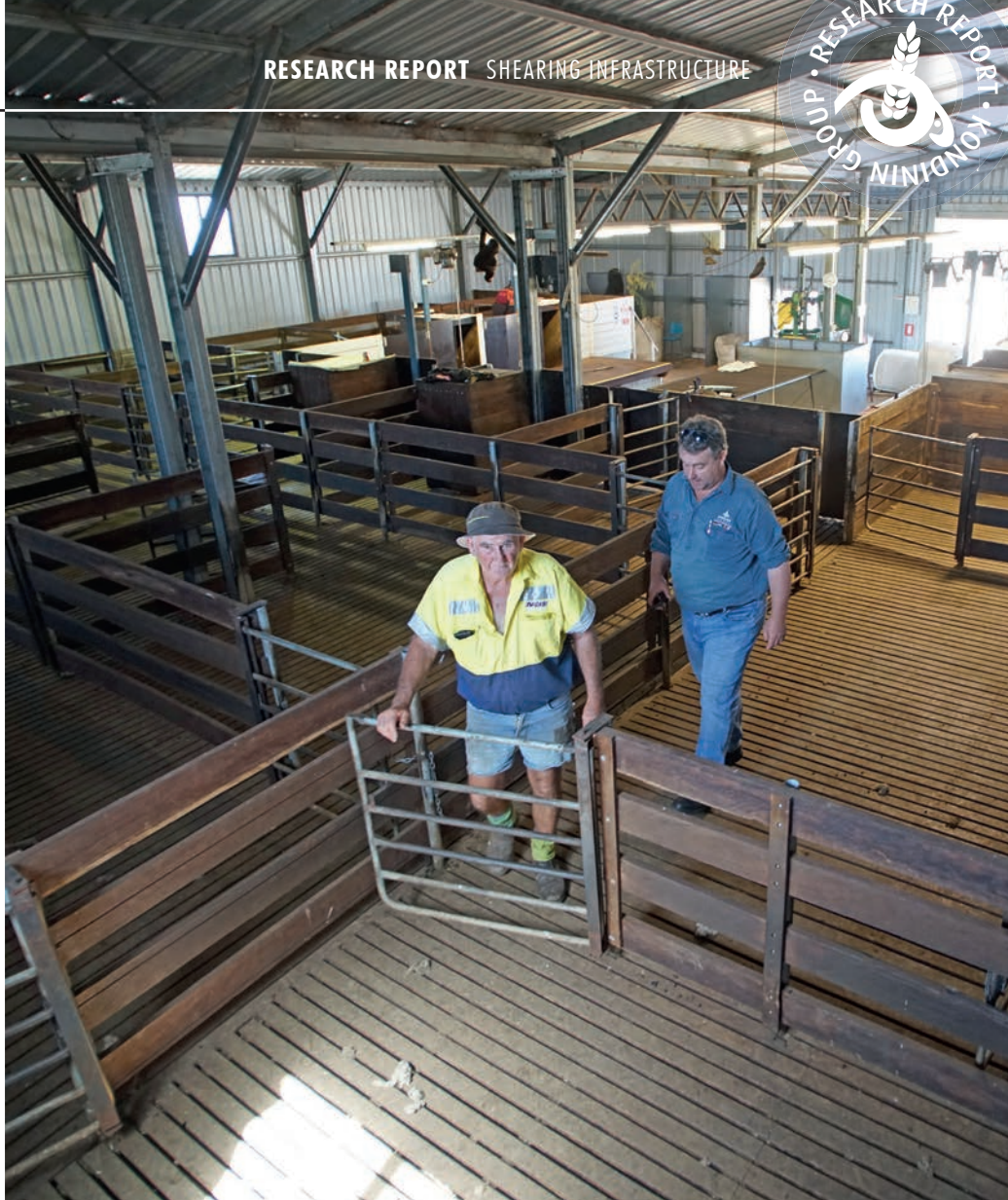
Don built all of the gates from steel offcuts. Gates slide through to aid when penning-up.
