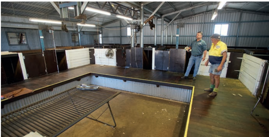
The six-stand, U-shaped board is arranged so the shed hands are no more than one step from the table at all times. Note the yellow line to improve the visibility of the edge of the board.
