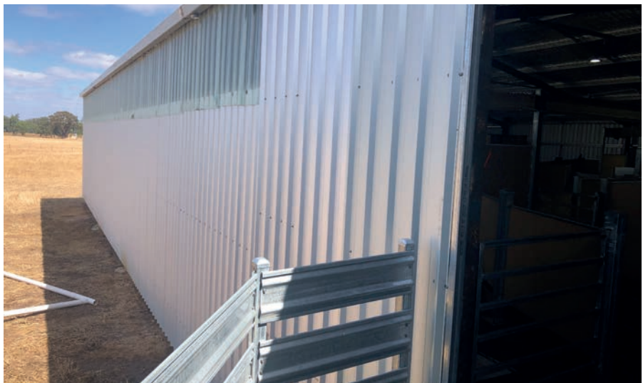
Let there be light: The new shed includes clear plastic sheeting to improve lighting conditions in the shed.
