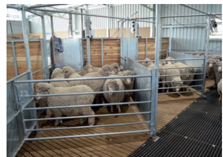
Fancy floor: Flooring has a mix of timber slats and plastic square grating.
