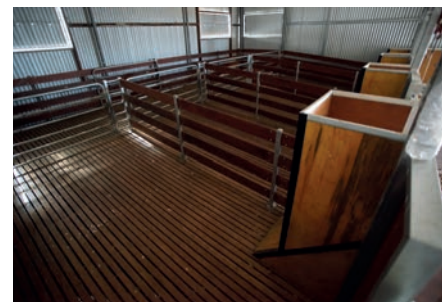
Sheep are forced directly from the raceway into the four catching pens. The catching pens have a sloped floor but the raceway is level. Sheep enter the raceway up a ramp from the right.
