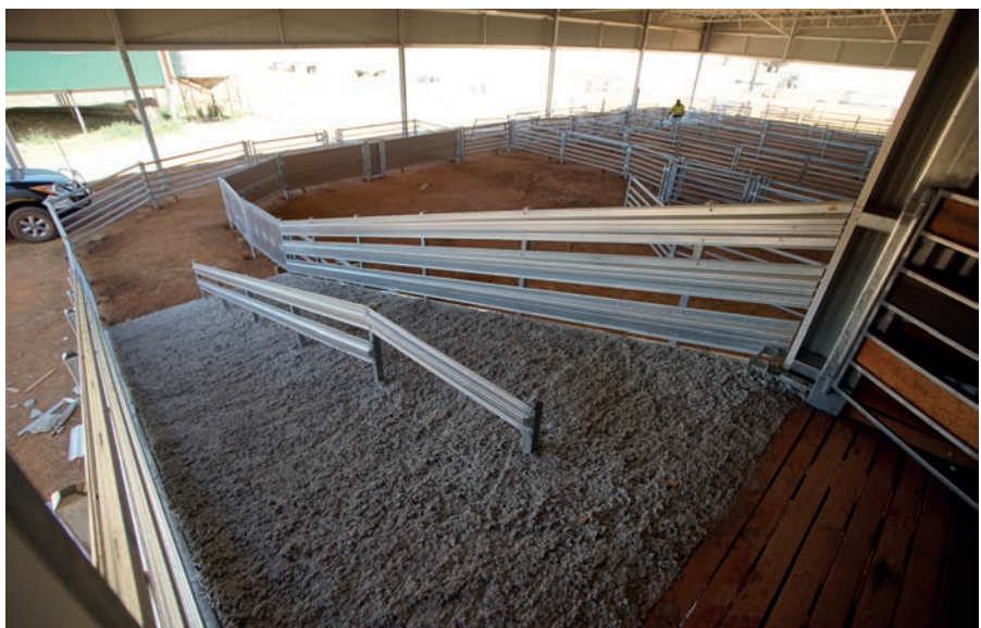
Ramp it up: Rough-pour concrete up-ramp into the shed with a half-height fence to stop sheep turning.
