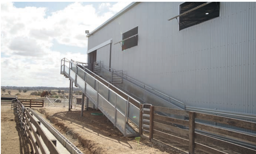
Ramped: Given the elevation of the floor, a long ramp is required to get sheep into the shed, but with blank walls and a parallel catwalk for personnel, the sheep flow up the ramp and flood the shed smoothly and quietly.
