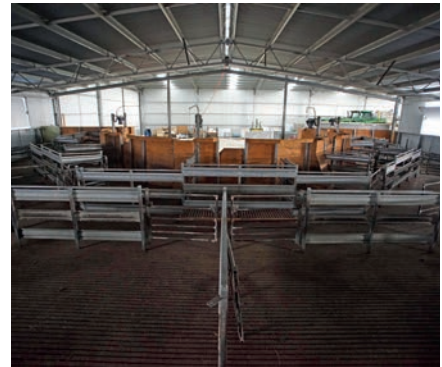
Front fill: Catching pens have a sloping floor and holding pens run parallel to the horseshoe design of the board.
