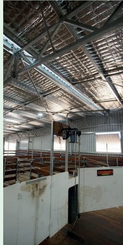
Ridge cap vent and insulation: Vented top caps and insulated roof: Insulation minimises radiated heat from the roof on hot days and condensation dripping off roof sheeting on cold mornings while the vented top cap provides heat flow out of the shed and work well with pivoting windows. Air conditioning (evaporative) has also been installed in some sheds to supplement ventilation cooling.
