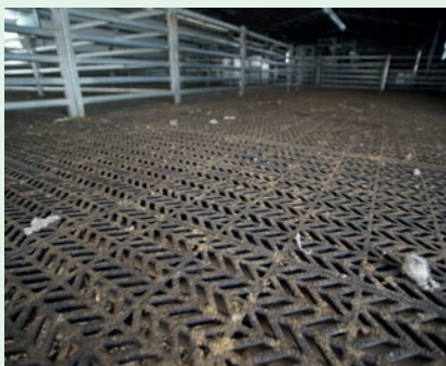
Plastic floor grating: While it looks like it would clog up, it clears freely is quiet and the modular design can be cut to replace old slat flooring. Not to be used in the catching pens however where it is too grippy. Comes in 1200x400x40mm interlocking sheets costing around $40/sheet or ($83/m 2 ).
