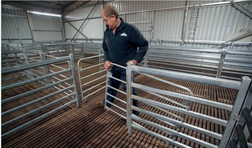
Slide swing gates: Used when flood-filling a shed and means gates can be closed without the wide clearing required for a simple swing gate. Available in prefabricated form in a range of widths.
