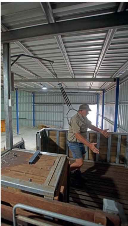
Catching pen door placement and lack of overhead structure allows the shearer to enter the pen while still wearing their back-aid.
