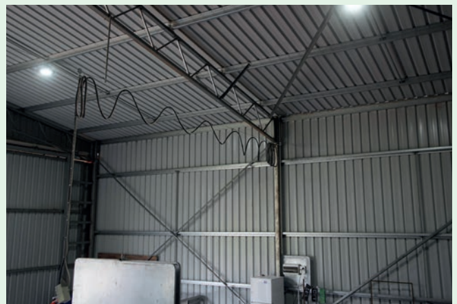
Power: USB outlets for charging phones and plenty of power outlets for radios and accessories. Power cords for the wool press suspended from high wires or on swing-away arms to keep them out of the way and allow the press to be moved.
