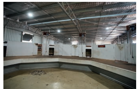
Cool feature: An insulated roof with vented ridge capping ensures temperatures in the shed during February are more comfortable.
