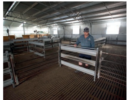
Steel yards: Galvanized K-rail style panelling with an RHS top member provides plenty of height for large framed sheep.
