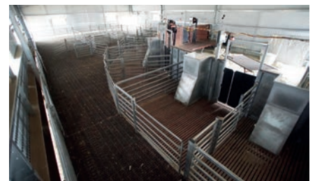
Materials: Plastic flooring, with timber board and catching pens, plastic catching pen doors and galvanised steel pens and holding yards round out the materials list.
