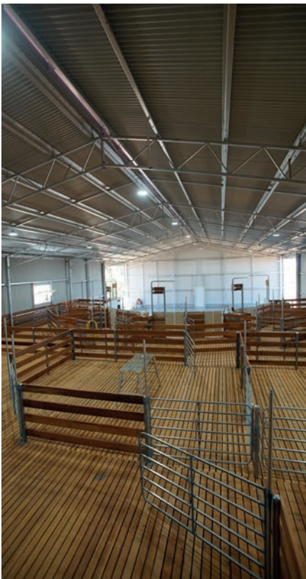
Flooring: Wider than normal (40mm) Karri grating installed with counter-sunk hex-head fasteners.
