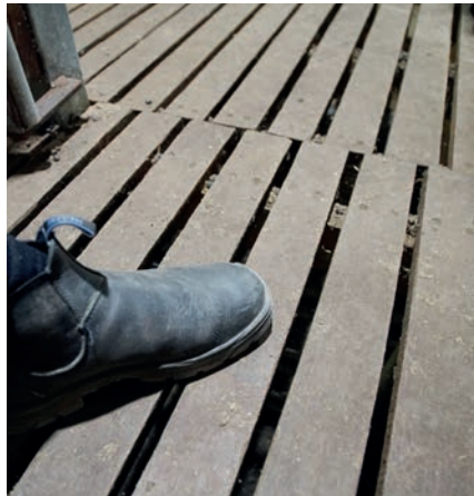
Don uses jarrah slats milled on the farm. The slats are wider than normal and are spaced at about 16mm.
