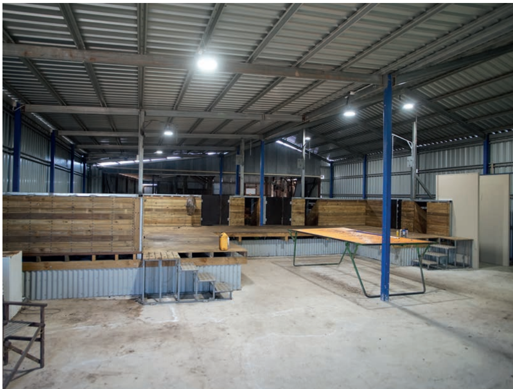
The four-stand shed has just been completed. Both sheds took Don about 12 months to build it in between other farm work.
