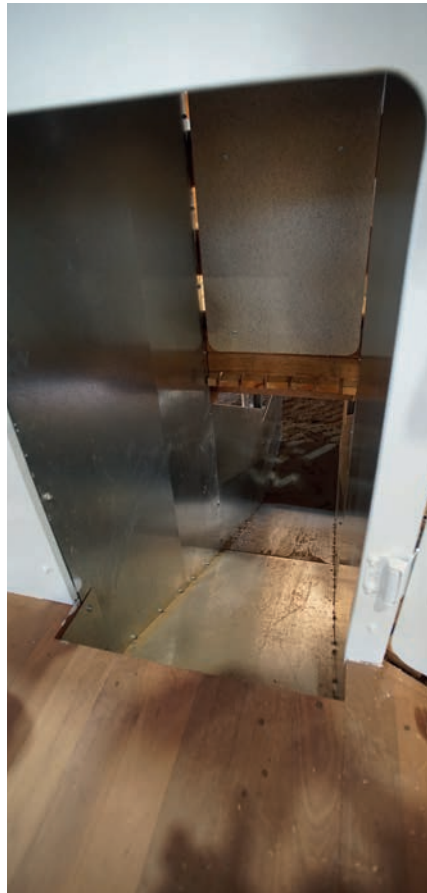
Chute transition: A recessed board and 200-300mm drop down into the chute.
