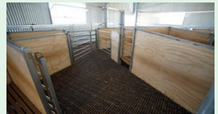
Ply and chipboards use: Ply and chipboard use is increasing including catching and holding yards.
