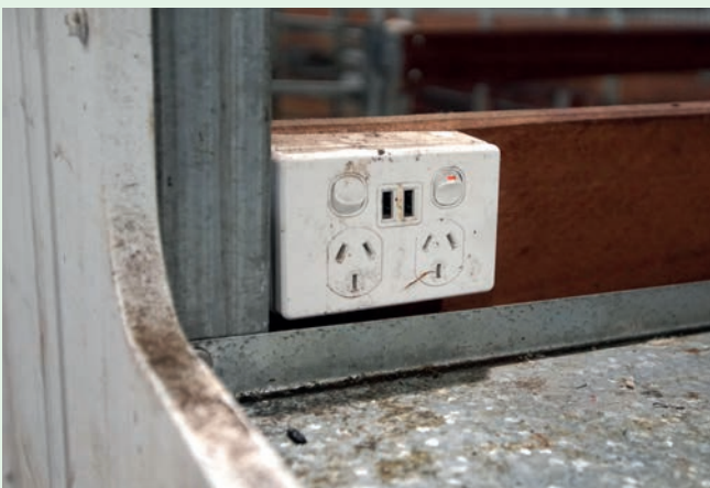
Power: USB outlets for charging phones and plenty of power outlets for radios and accessories. Power cords for the wool press suspended from high wires or on swing-away arms to keep them out of the way and allow the press to be moved.
