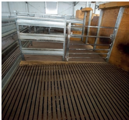
Sloped: Only the catching pens slope toward the board, rising up from the main floor level.
